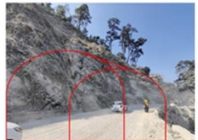
Road stretch of proposed cut and cover section at rock slide zone
