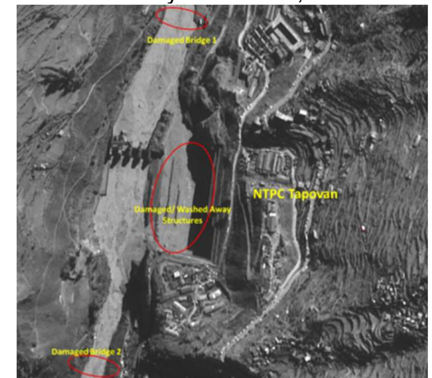
Damage to Tapovan Project due to flash flood in Rishi Ganga River, Feb 2021
