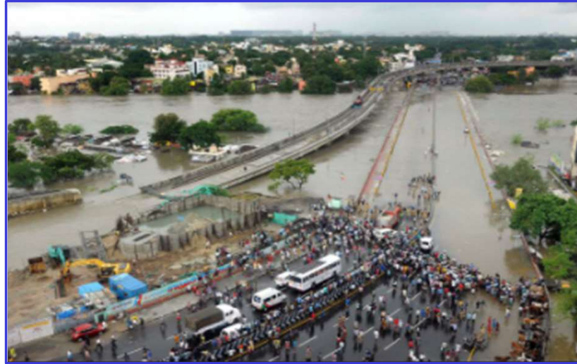
Maraimalaiadigal Bridge, Saidapet
