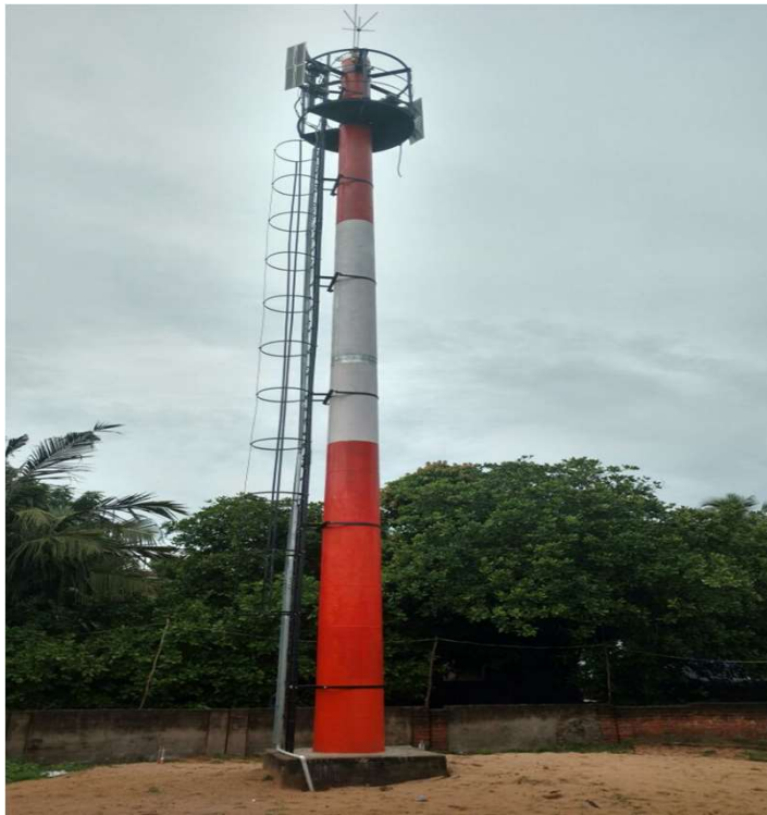
EWDS Tower, Ganjam, Odisha
