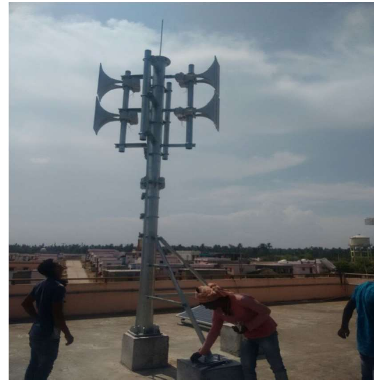
EWDS Tower installed on the roof top of MPCs, Ganjam, Odisha
