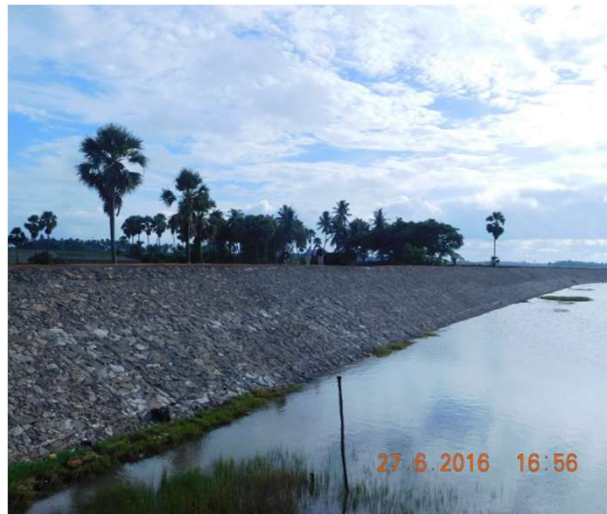
Saline Embankment, Keutajanga Block, Puri Dist., Odisha
